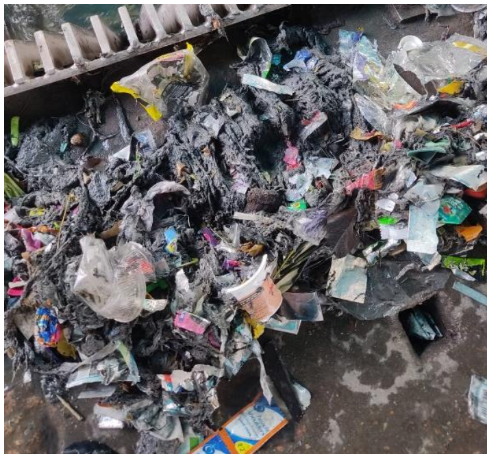
Figure 18. Screen chamber debris containing fleshes and hair in preliminary treatment at STP Jajmau
