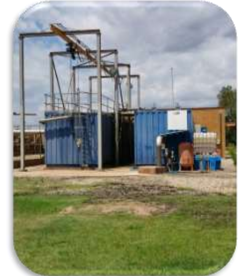
MBR effluent, Spain
