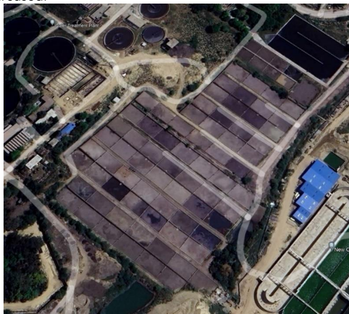
Figure 6: Existing sludge drying beds at STP Jajmau, Kanpur
