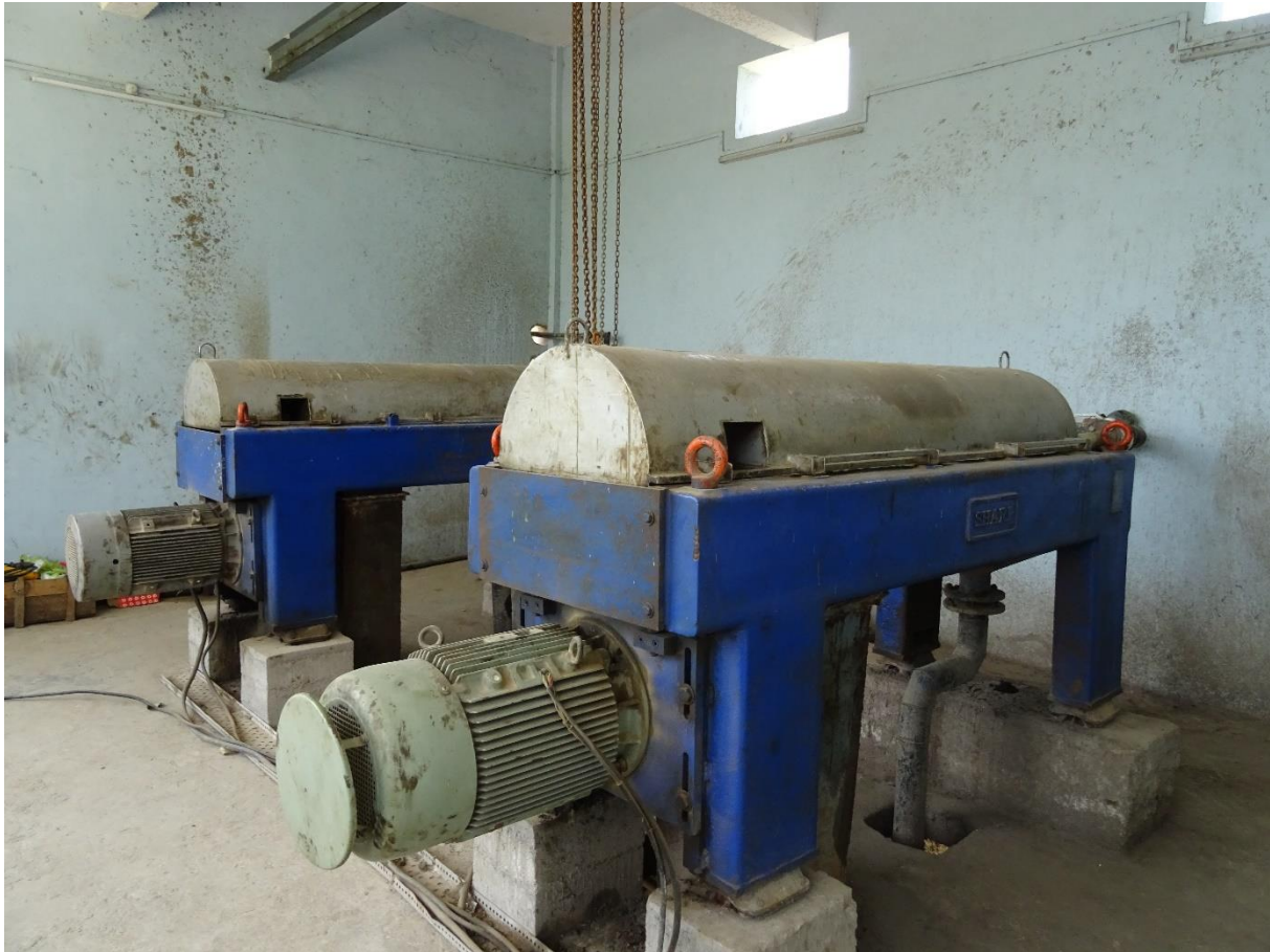
Figure 21: Sludge dewatering Line 2
