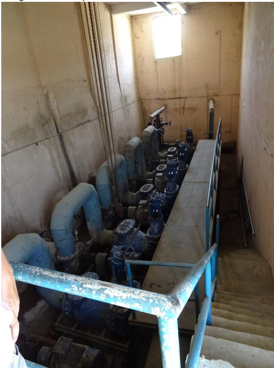
Figure 19: Effluent pumping station Line 2
