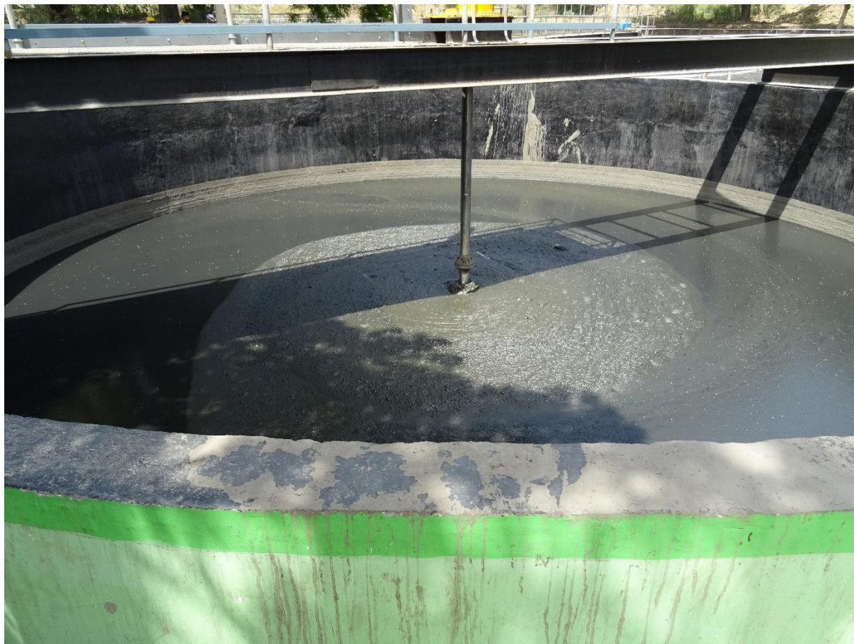
Figure 11: Sludge blending tank Line 1
