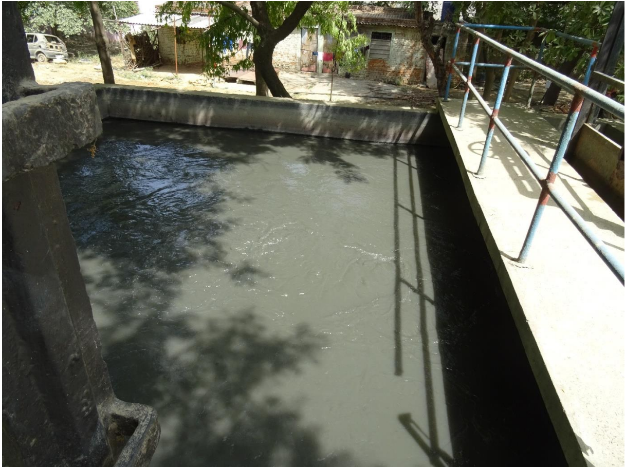
Figure 4: Inlet reception tank
