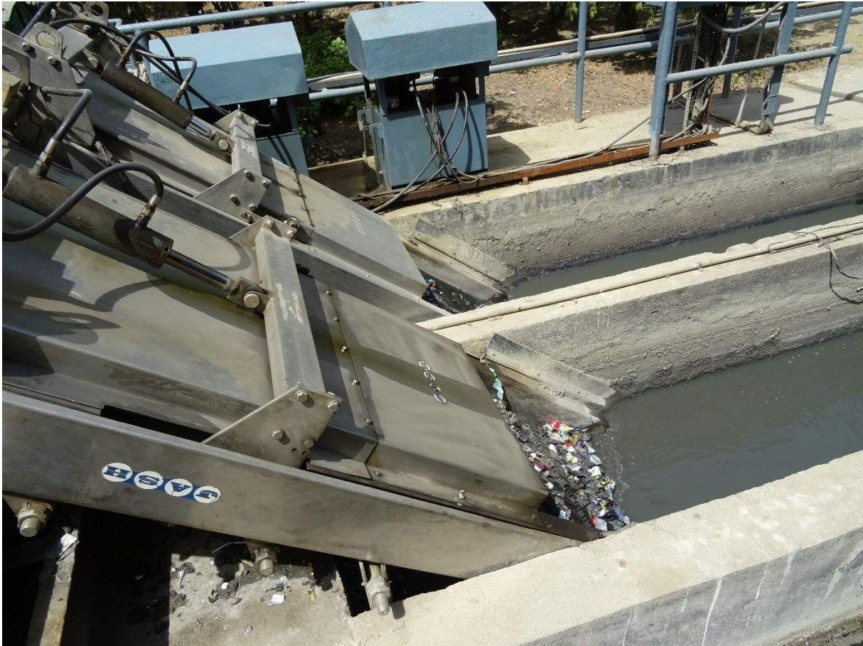
Figure 13: Inlet screens Line 2
