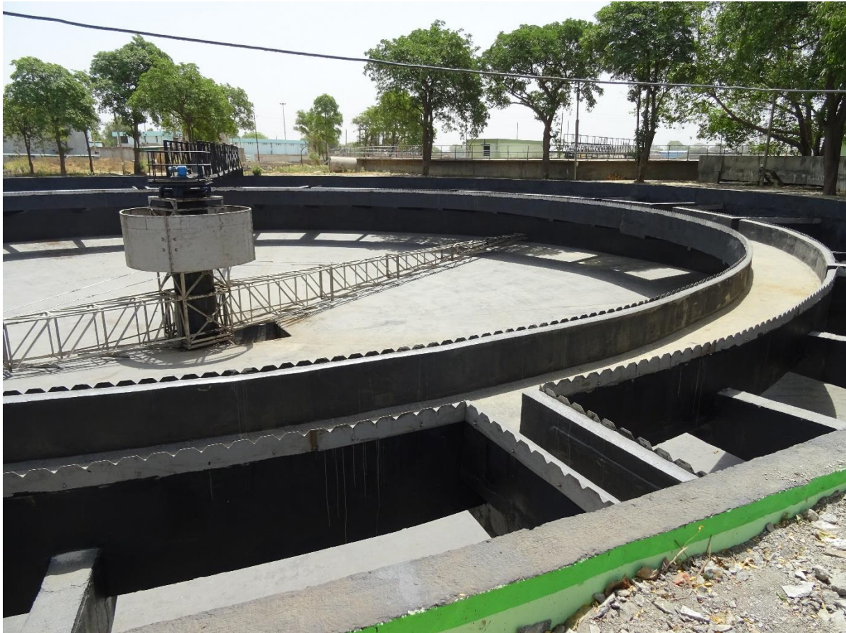
Figure 10: Renovation in progress on the secondary clarifiers of Line 1
