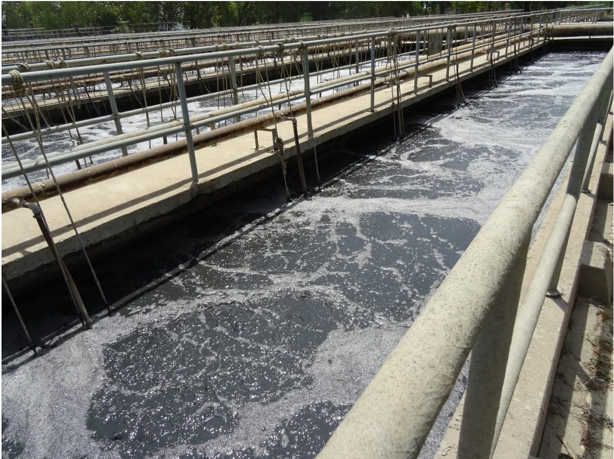
Figure 17: Aeration tank Line 2
