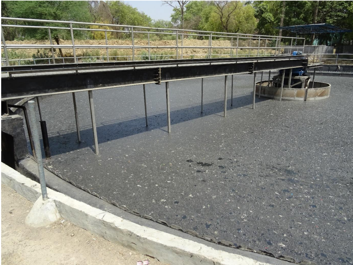
Figure 12: Sludge thickeners Line 1
