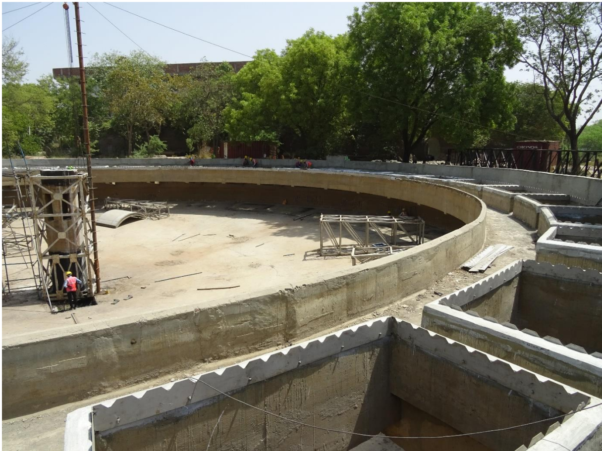
Figure 8: Renovation works in progress on primary clarifiers Line 1
