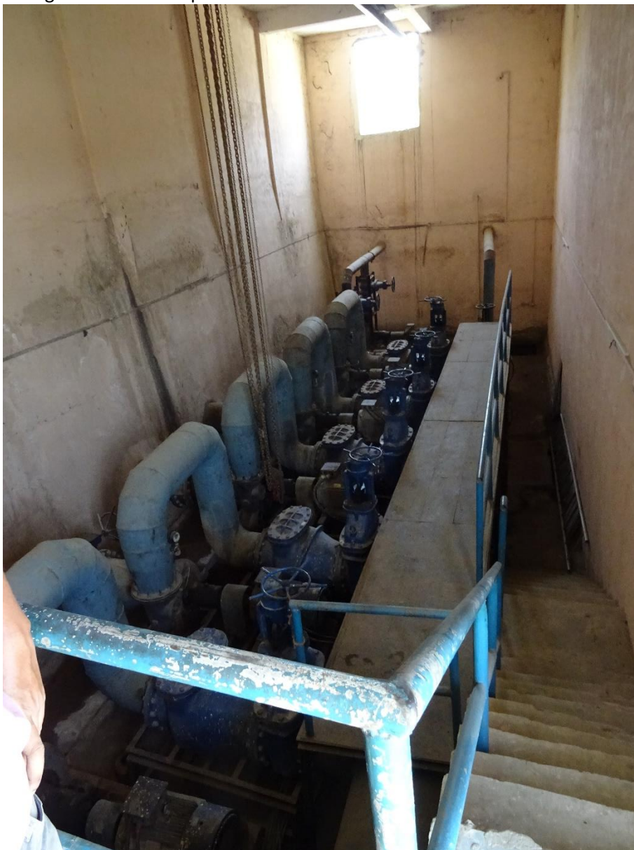
Figure 19: Effluent pumping station Line 2
