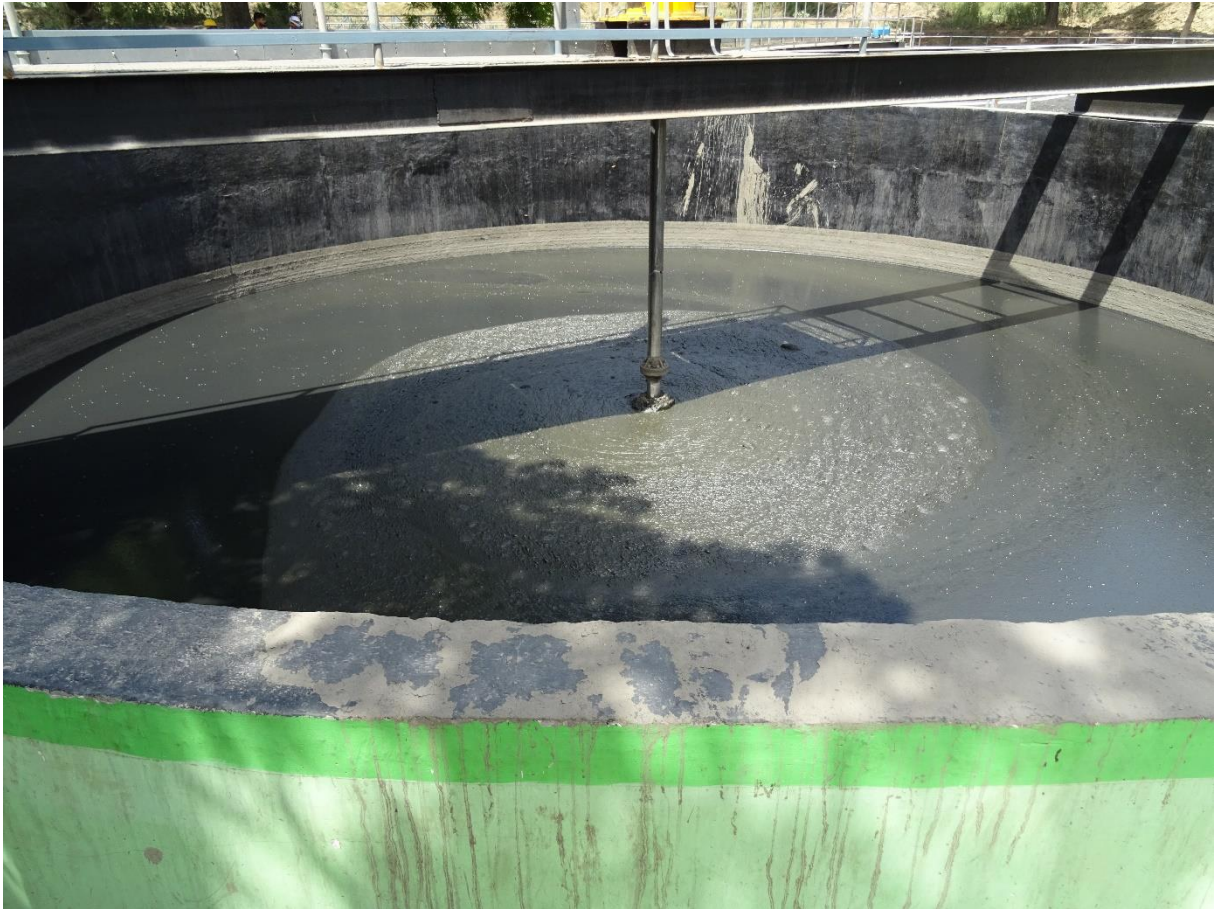
Figure 11: Sludge blending tank Line 1
