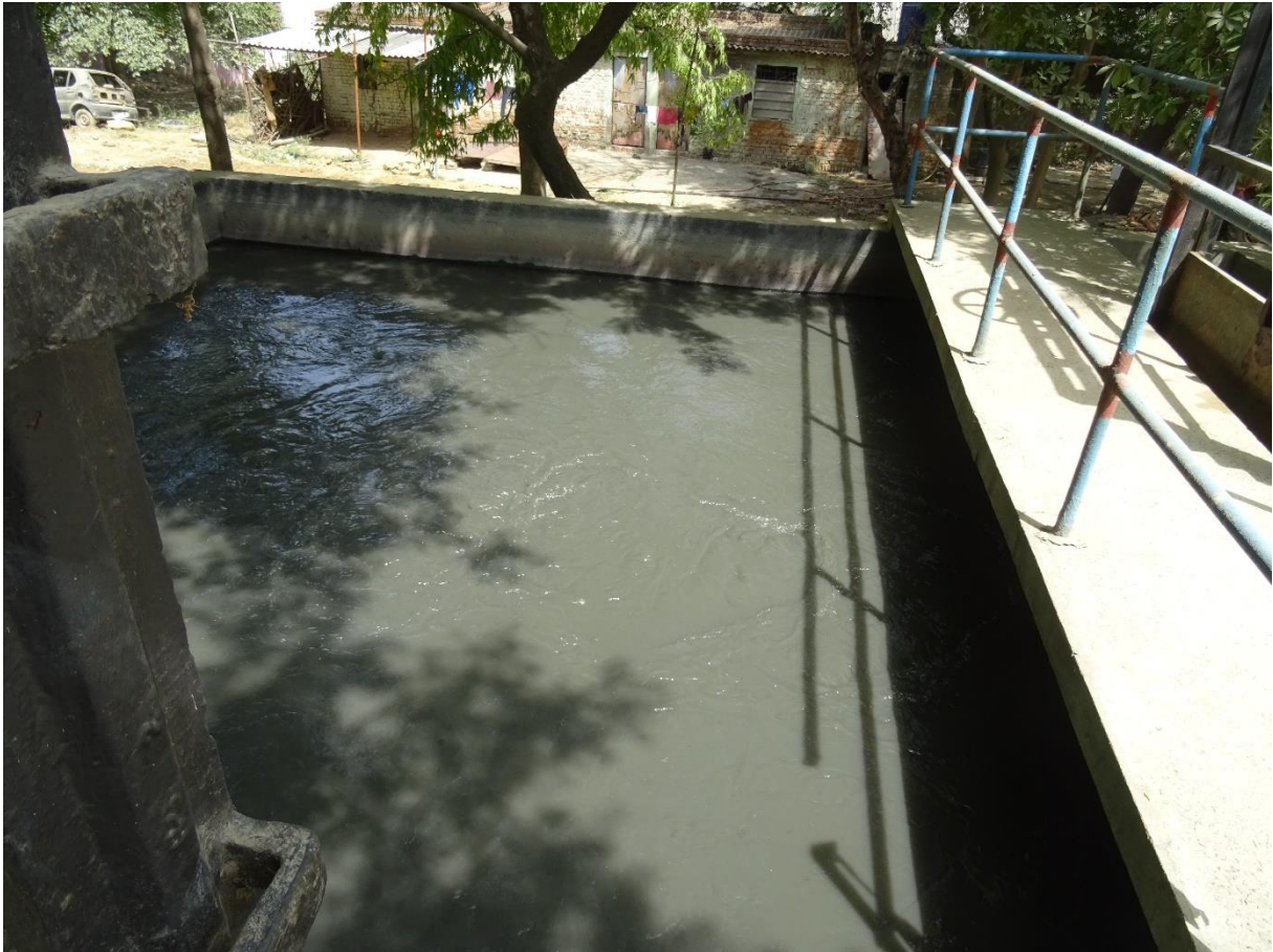
Figure 4: Inlet reception tank
