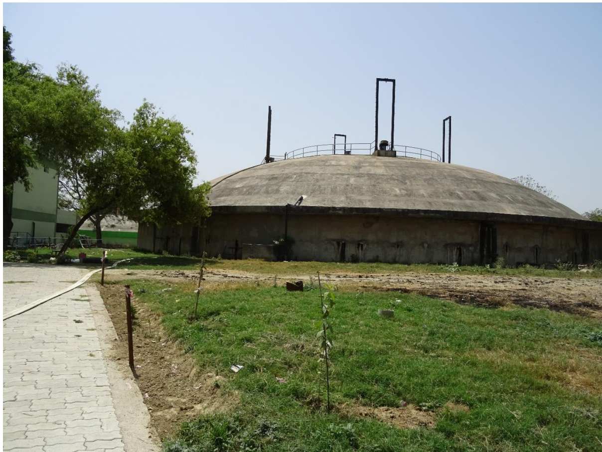
Figure 20: Sludge storage tank Line 2
