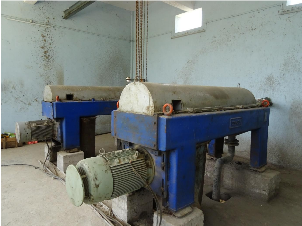
Figure 21: Sludge dewatering Line 2
