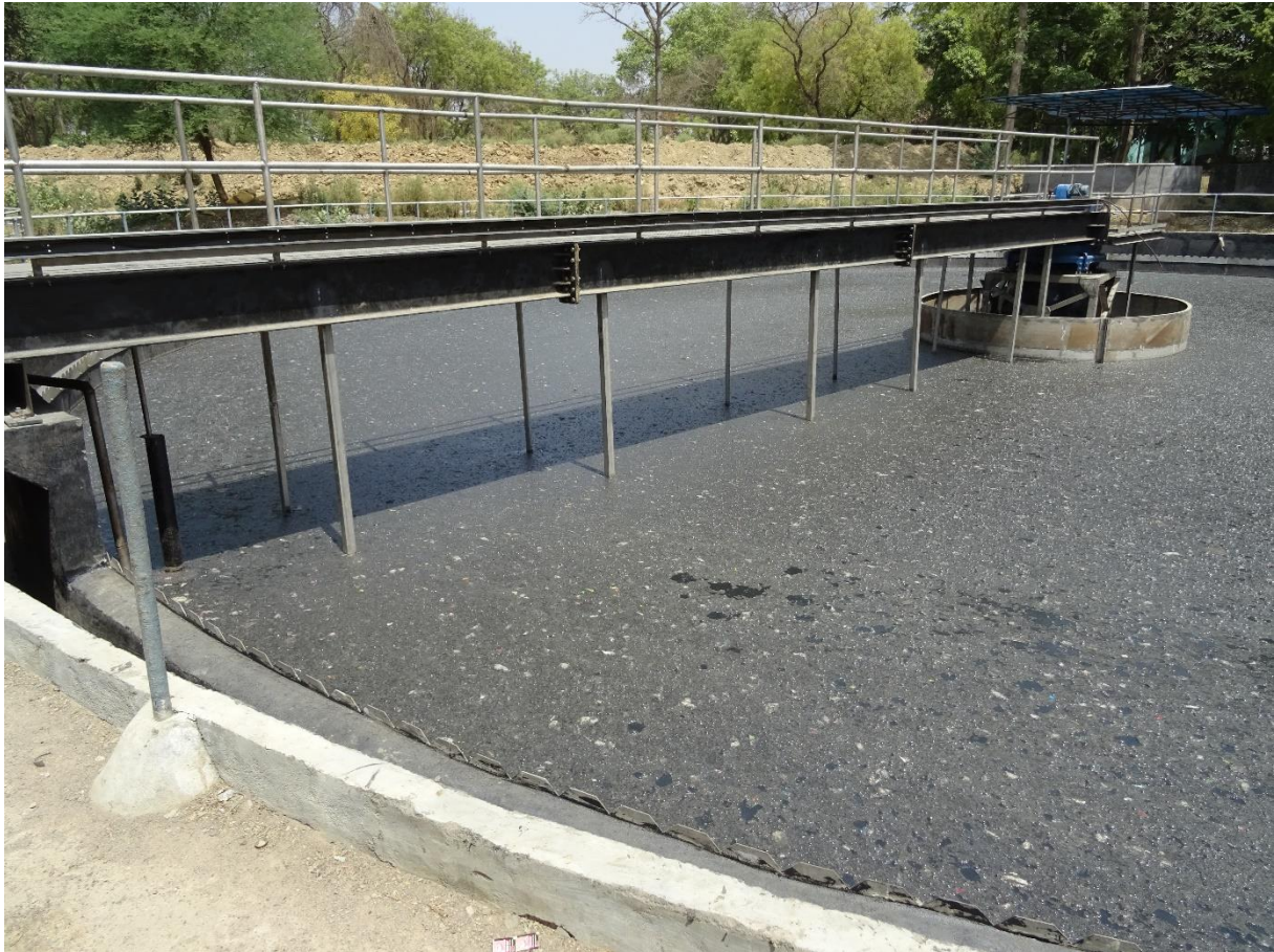
Figure 12: Sludge thickeners Line 1
