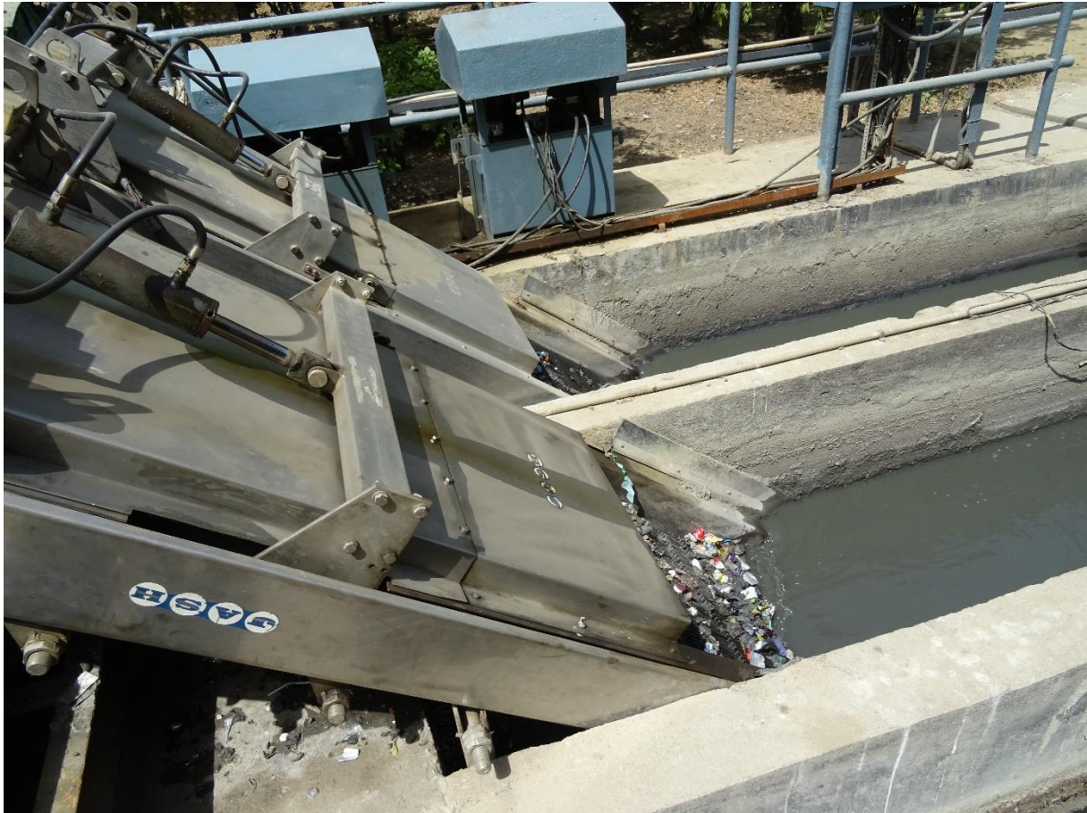
Figure 13: Inlet screens Line 2
