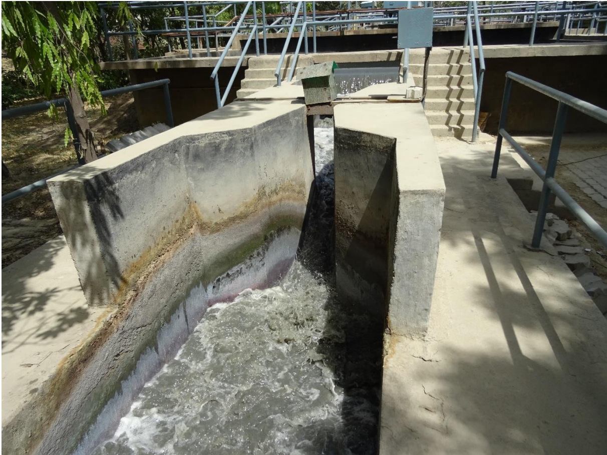
Figure 15: Inflow flume line 2
