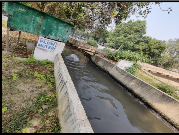
Raw Domestic Sewage
