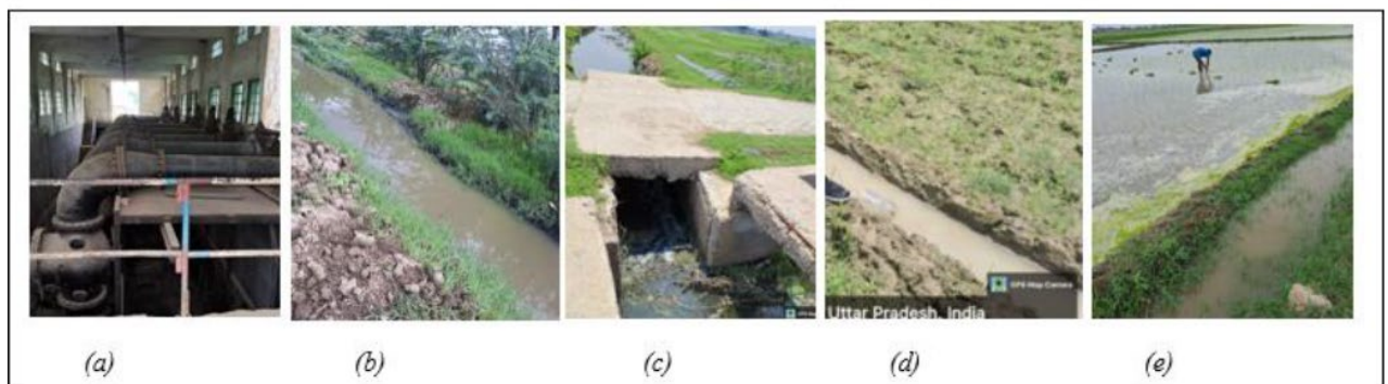
Figure 3: The flow of the effluent from the STP through the irrigation channels to the agricultural fields in the village (a) STP effluent pipes, (b)-(c) channels with effluent pipes, (d) irrigation channel next to the field, (e) effluent being used for flood irrigation (Babalola, 2022)
